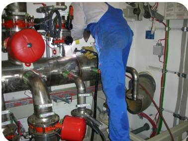
Working at the fitting.
